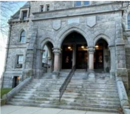
City Hall North Entry Lower Stairs
